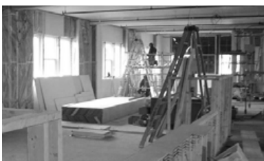
Renovations on the second floor of 97 Victoria St. N in 2006
