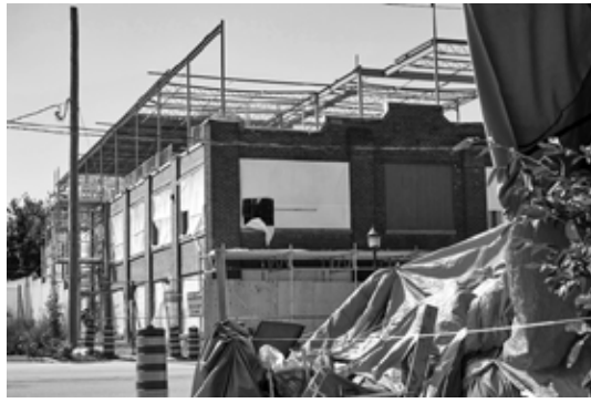
Construction on 97 Victoria viewed from the 100 Victoria St. encampment site
