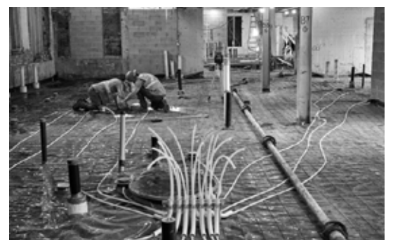
Workers installing plumbing and utilities on the ground floor level
