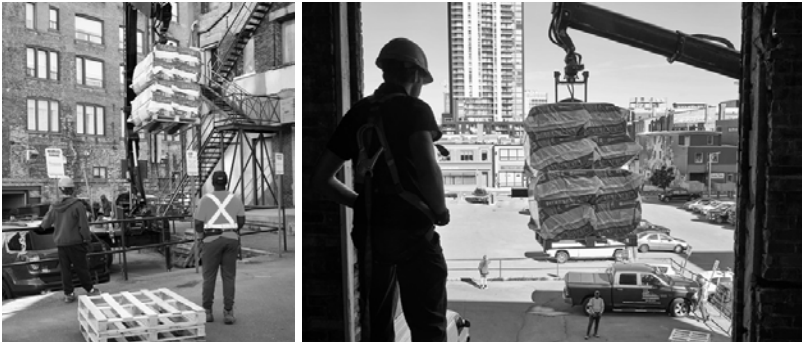
Above: Workers build the upper floor of a loft style unit; A small crane lifts materials up to the second and third floors
