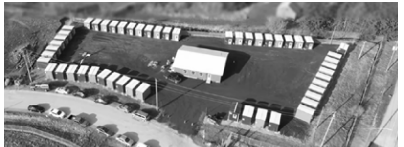
50 individual cabins and a central community building are located at the Erbs Road Shelter site at 1003 Erbs Road. Cabins include a bed, desk and chair, shelves, mini-fridge, and air conditioning unit
