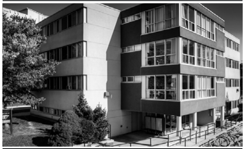
This year, The Region of Waterloo is providing funding for The Working Centre to convert an unused student housing building into interim housing for 80 individuals
